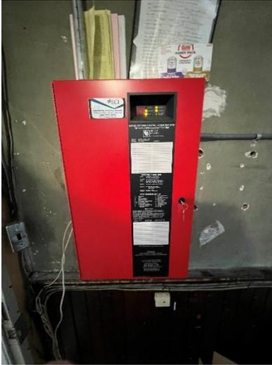
Figure 6.0 – Fire Control Communicator Box
