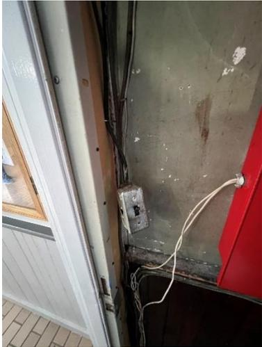
Figure 8.0 – Exposed wiring Mech. Room
