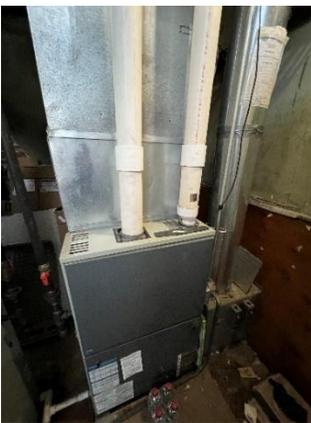
Figure 7.0 – Direct-vent Furnace
